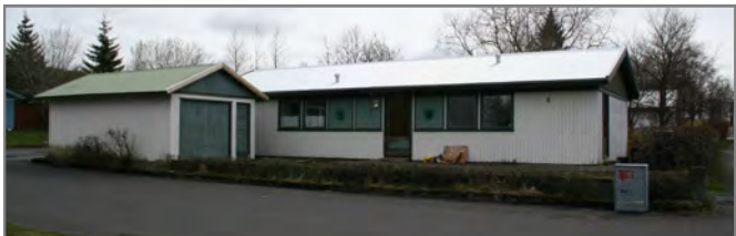
Lambastekkur 8, einingahús innflutt af FB
